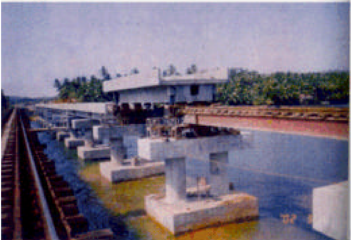
Line Boulding Project Bridge No. 1162 Along Calicut Mangalore
