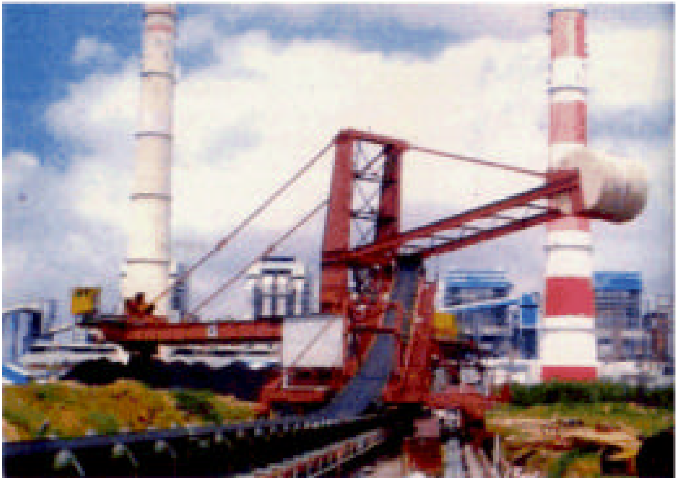
NTPC Talcher Stage-II (4x500MW) — Overall View
